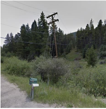
Existing Shadow Mountain Drive Overhead Powerline Corridor
