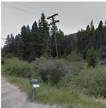
Existing Shadow Mountain Drive Overhead Powerline Corridor
