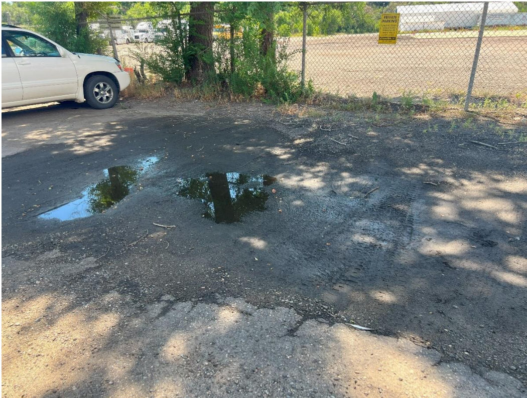
Figure 14. Unpaved Parking Lot
