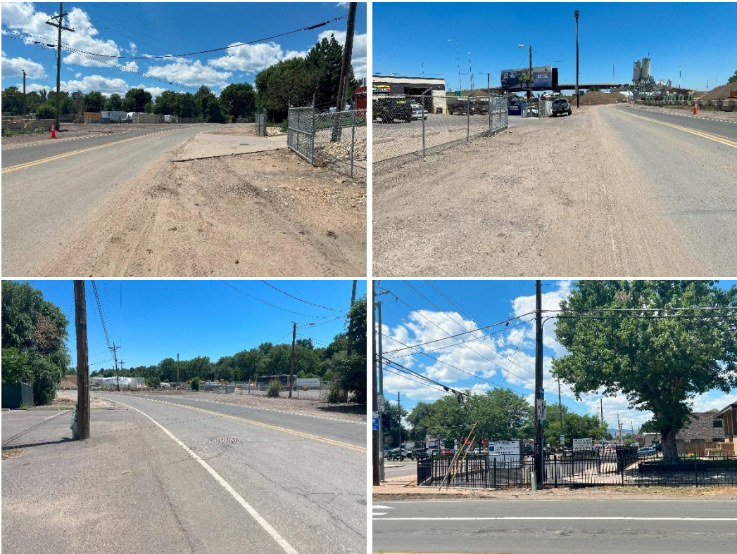
Figure 16. Lack of Pavement, Curbs, and Sidewalks
