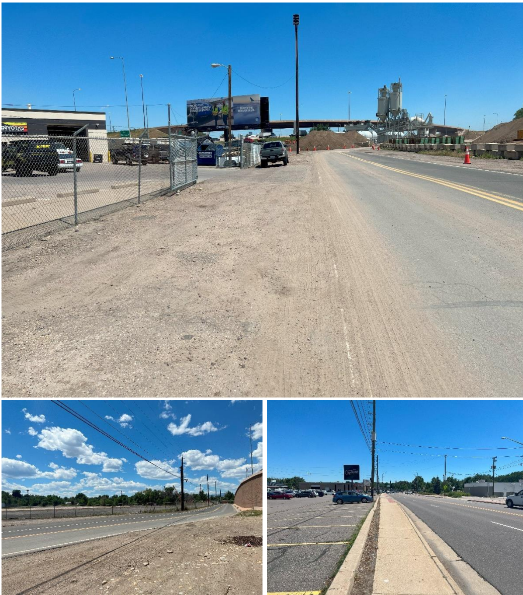
Figure 17. Presence of Overhead Utilities and Billboards
