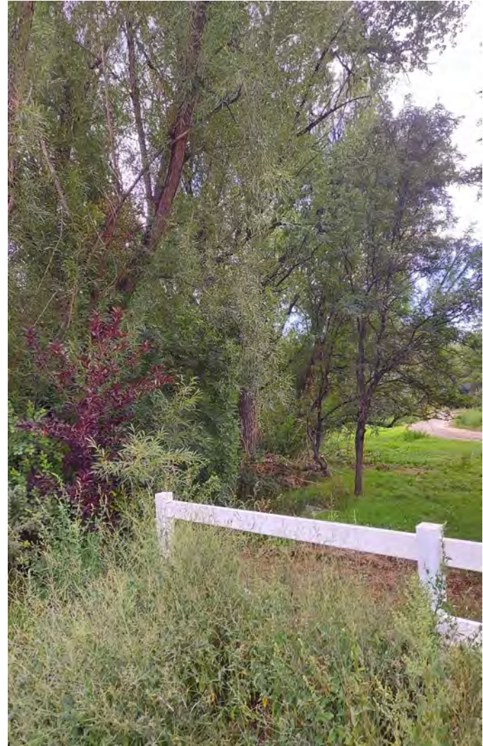
Photo 6. View of Raccoon Creek entering the northern boundary of the site from a culvert under West Leawood Drive, facing south
