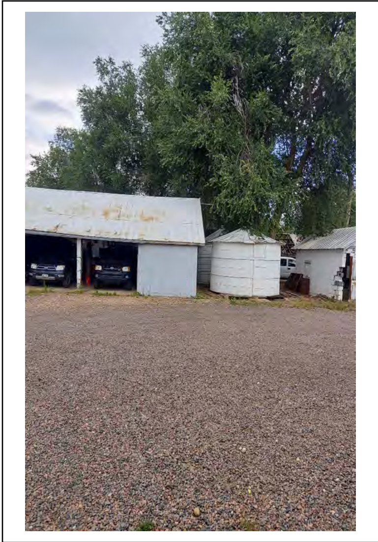
Photo 3. View of outbuildings and gravel driveway, facing north
