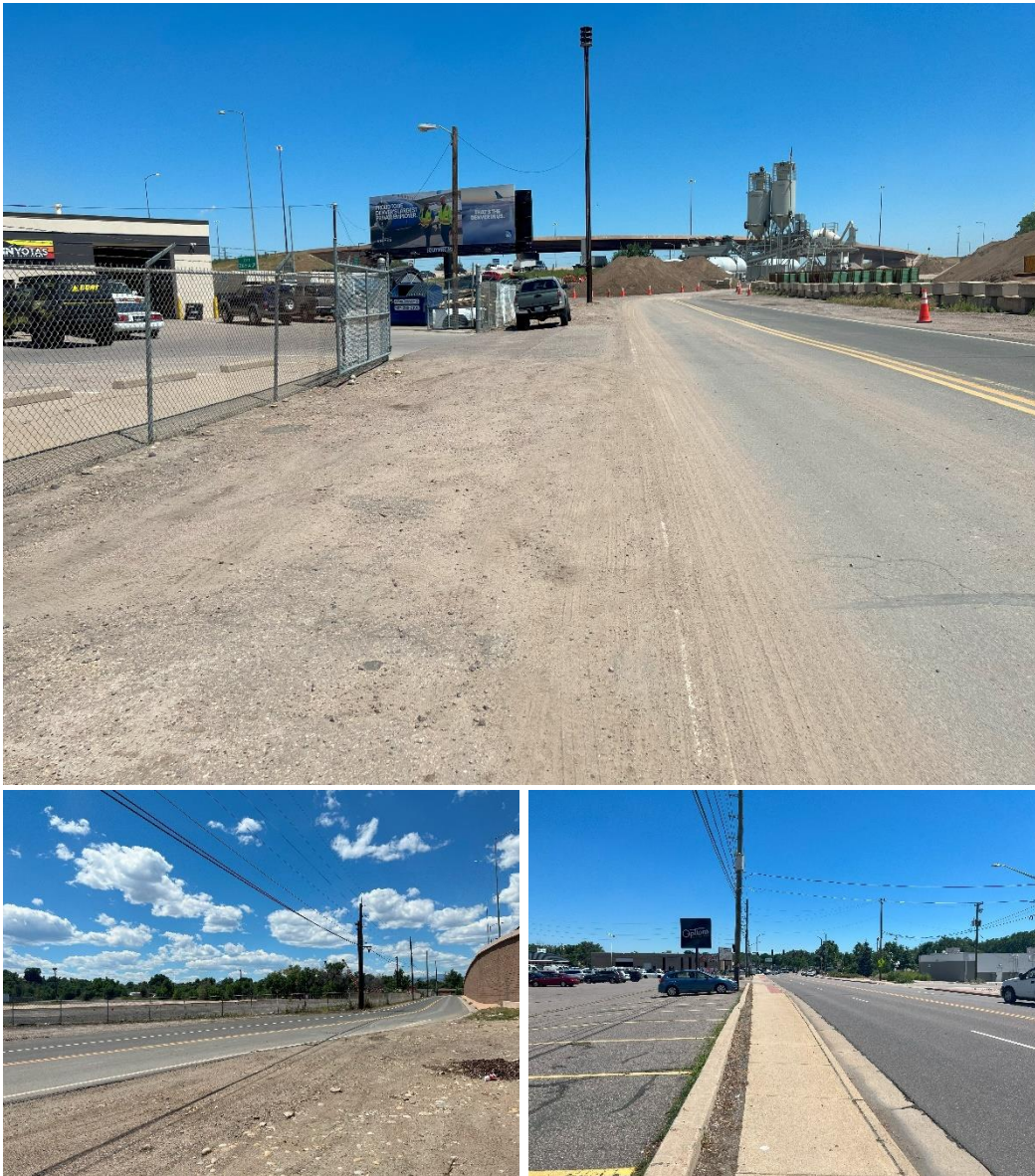
Figure 17. Presence of Overhead Utilities and Billboards
