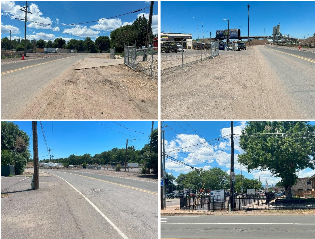
Figure 16. Lack of Pavement, Curbs, and Sidewalks
