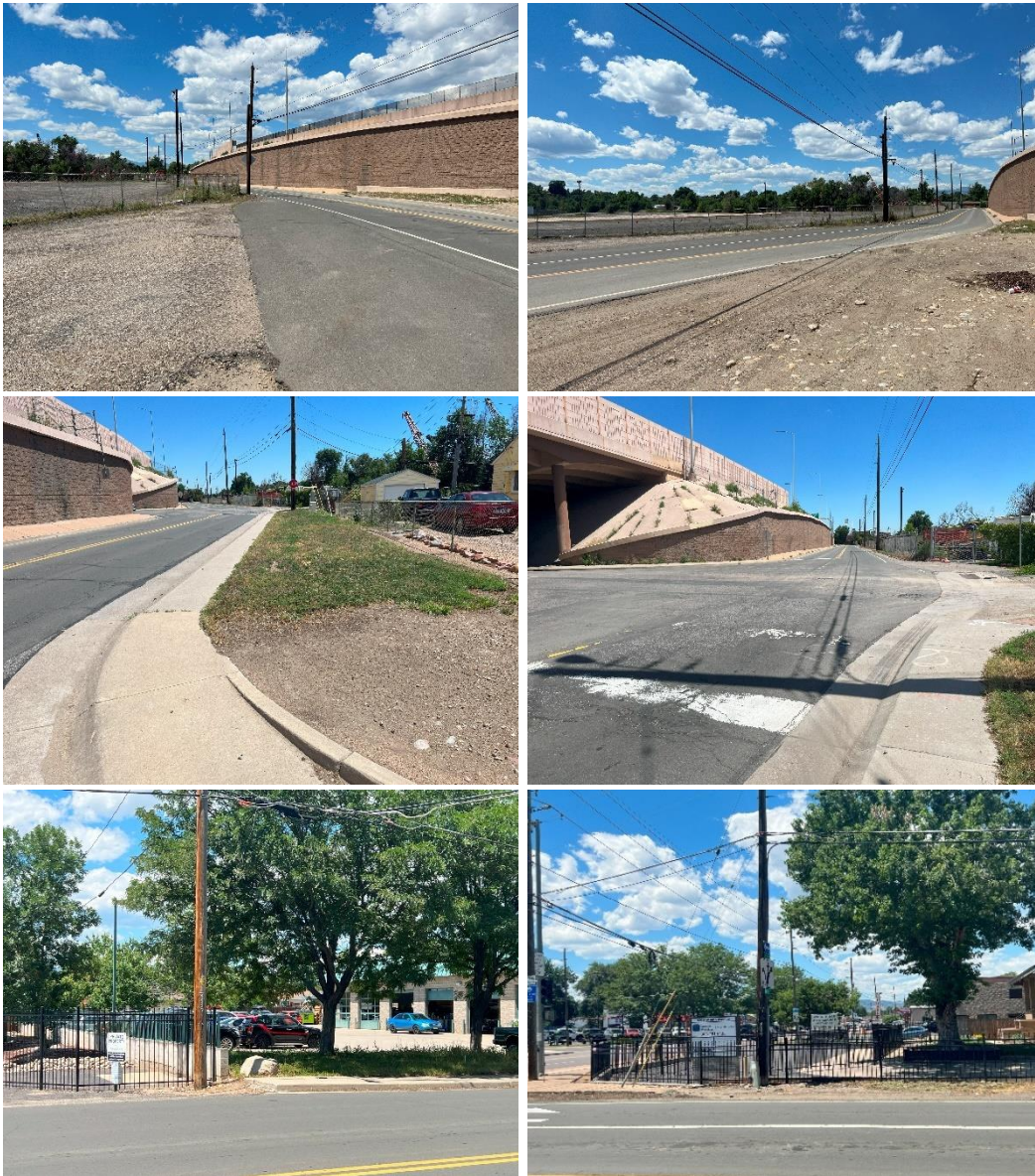
Figure 3. Poor Provisions or Unsafe Conditions for Pedestrians
